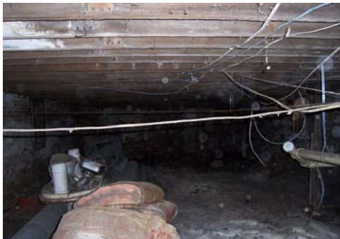
crawl space before retrofit
