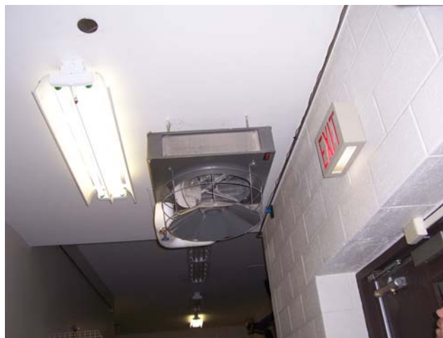
Figure 5.1 Ceiling Mounted Unit Heater
